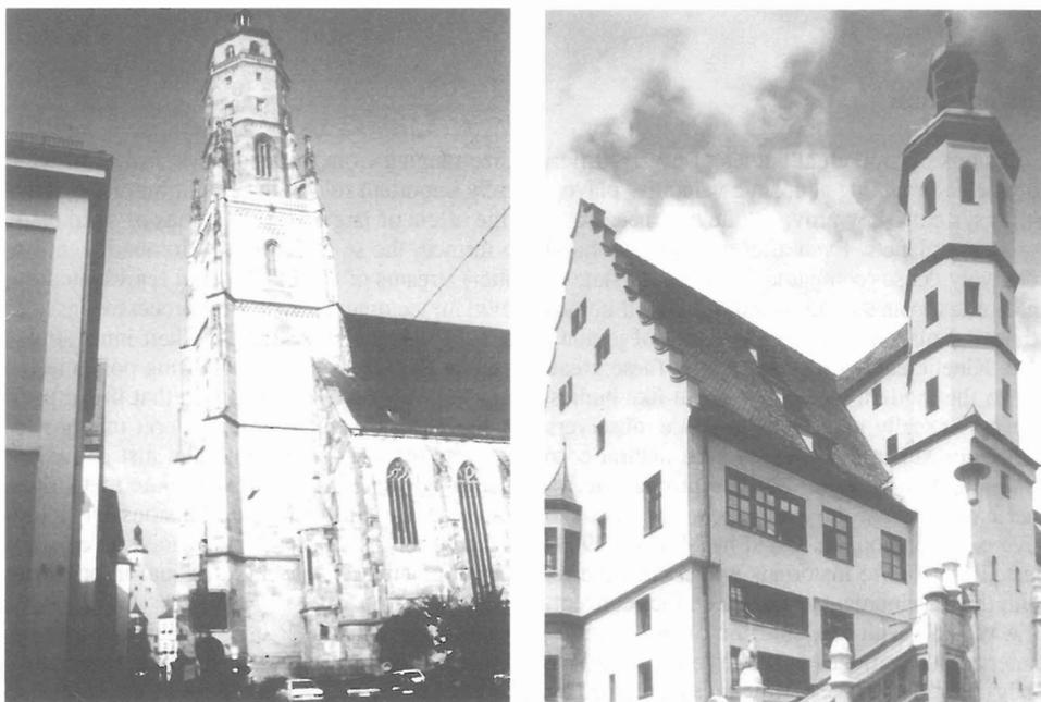
**Fig. 1. St. John's Church (a) and City Hall (b) in Nördlingen, Germany, built of suevite - an example of the use of local impactite for building purposes.**
