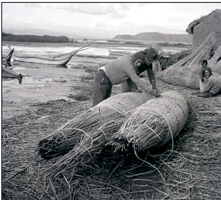
Pl. 21. Construction of a balsa reed boat, Suriki, Bolivia. Václav Šolc, 1963. Roll film negative 60 × 60 mm, Inv. No. Am I 1489.
