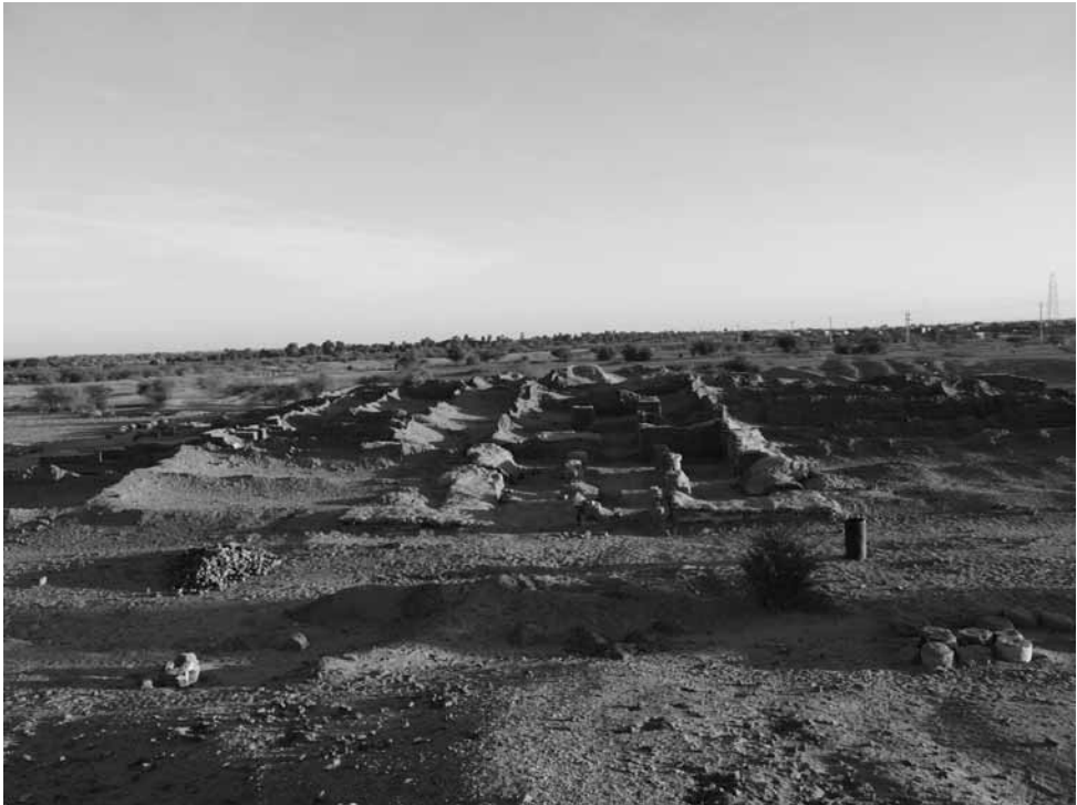
Pl. 8: View on the southern part of the Palace of Amanishakheto (Photo by Pavel Onderka).
