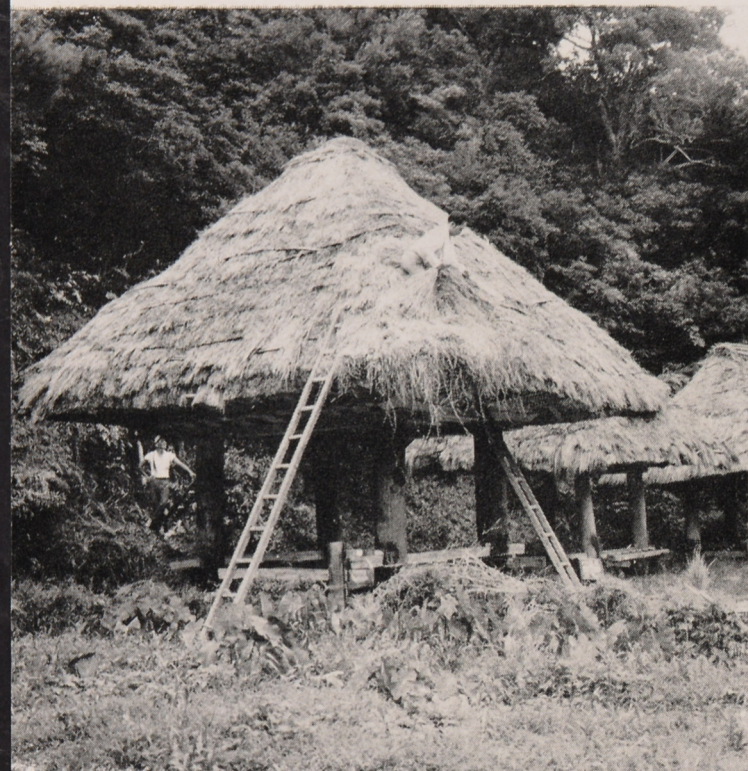
17: Repair of straw thatching on takakura . Kagoshima prefecture, Amami Ōshima, Yamato-mura.
