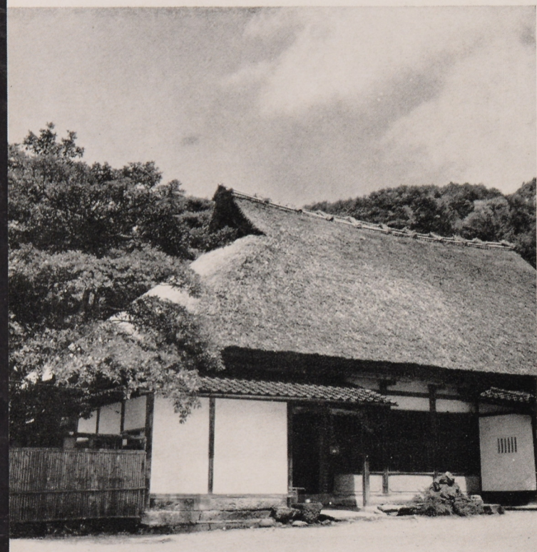
1: Tokikuni-ke, the house of the Tokikuni family, Ishikawa prefecture, Notō peninsula, Sosogihama.
