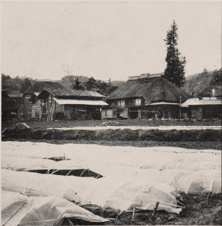
11: An interesting example of kiritoshi-yane . Basically the roof is in the yosemune shape but from both ends of the ridge it slopes down in a shell shape. Decorative ridge of the hakomune type. Nagano prefecture, Azumi-gun, Azumi-mura.
