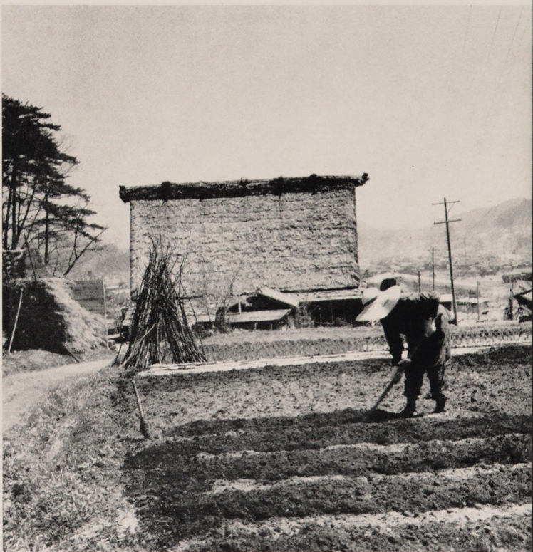
8: Side view of the roof of the gasshō-zukuri house from phot. No. 7.
