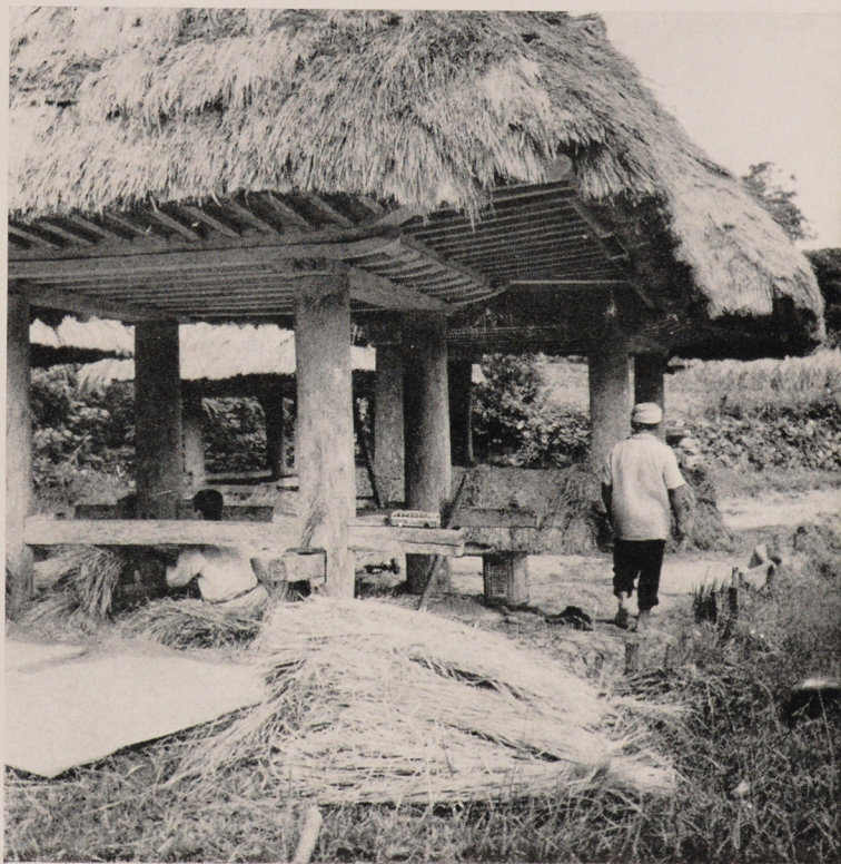
16: Takakura (high store-house), typical for the Ryūkyū islands. Kagoshima prefecture, archipelago Amami, Amami Ōshima, Yamato-mura.
