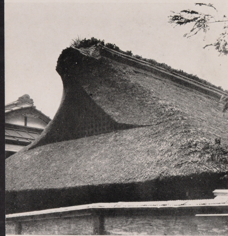
2: Detail of thatched roof of the irimoya shape. Tōkyō-to, Okutama, Mitake.
