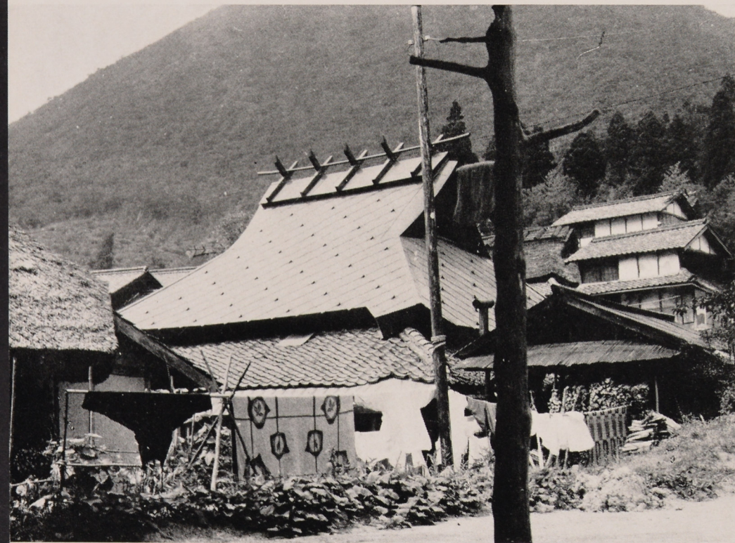
14: Thatched roof in the irimoya shape covered with sheet metal. The ridge decorated with rider ( noriuma ). Hyōgo prefecture, Tamba, Tachikui.
