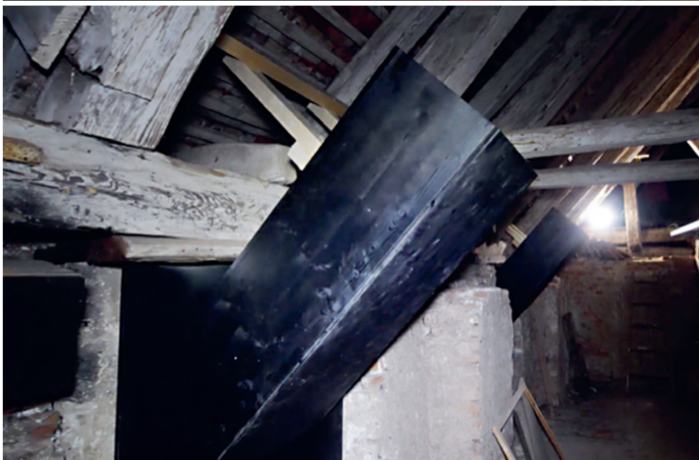
Figs. 2, 3. 2 (top) – Entrance to the chimney in the loft. 3 (below) – Entrance to the ducts in the loft.
