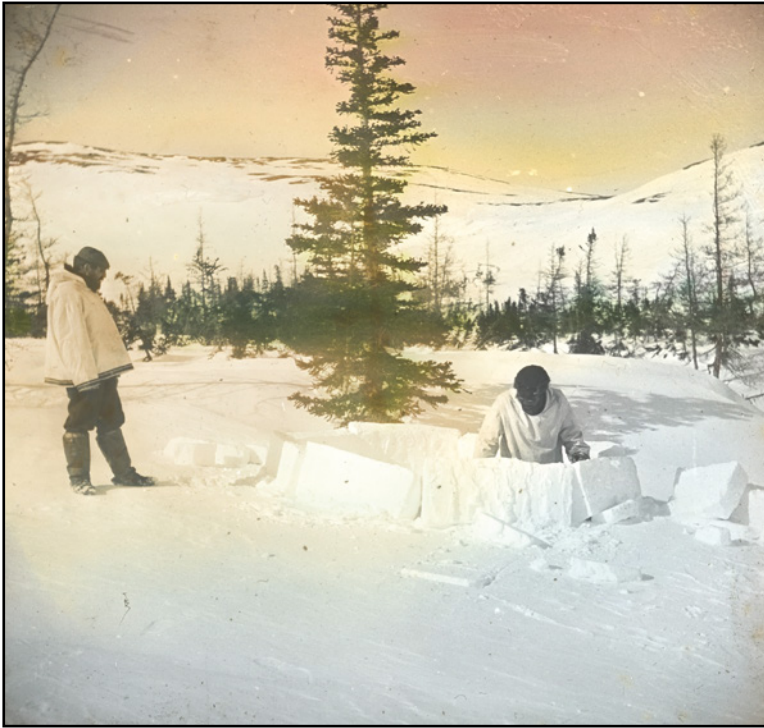
Pl. 24. Construction of a snow house. Canada, Labrador, coloured slide glass 85 × 85 mm, Inv. No. Am II 4188. (Photo: Jiří Jaeger, 1914–1919).
