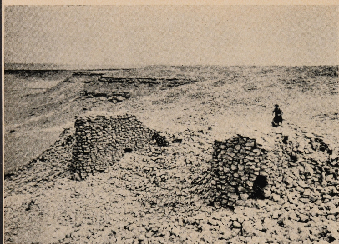
Fig. 3: Al-Xalqūm: protective wall.
