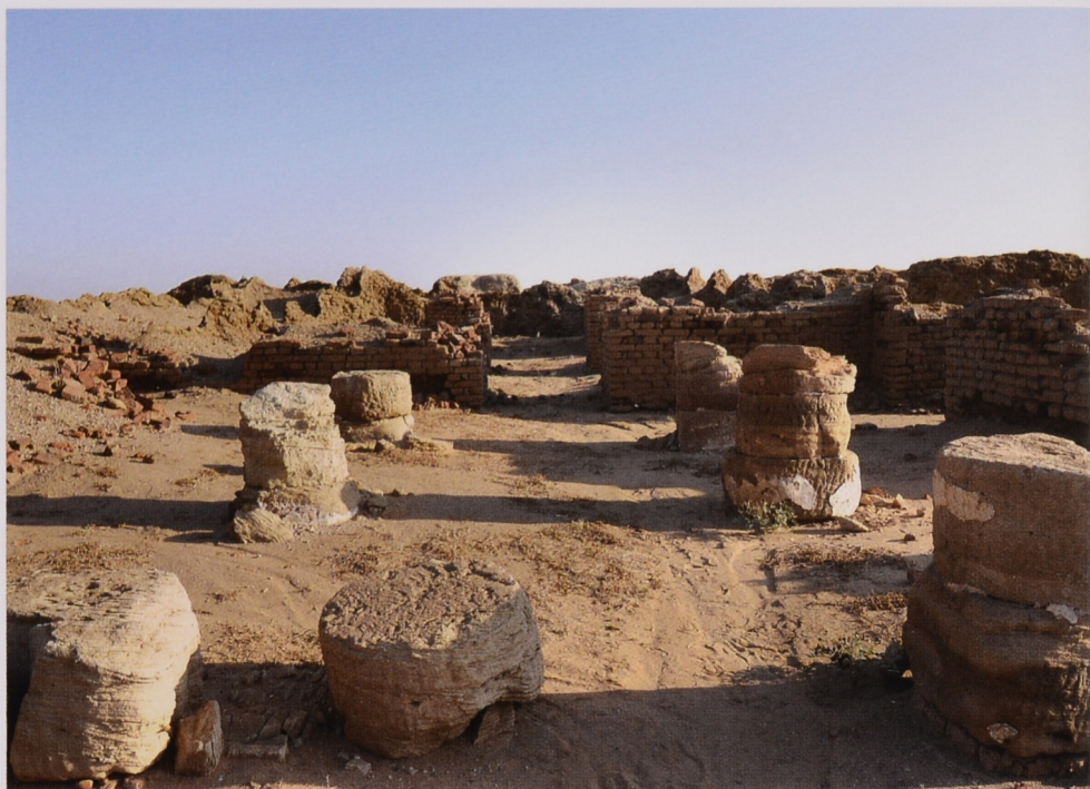
Pl. 7: The Southern Entrance to the Palace of Amanishakheto [photo by Pavel Onderka].
