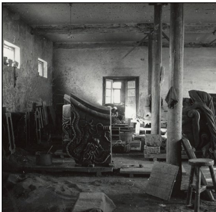
Pl. 5. Workshop for roof tiles making for the Forbidden City restoration, Beijing, China. Václav Šolc, 1957. Roll film negative 60×60 mm, Inv. No. As I 138.
