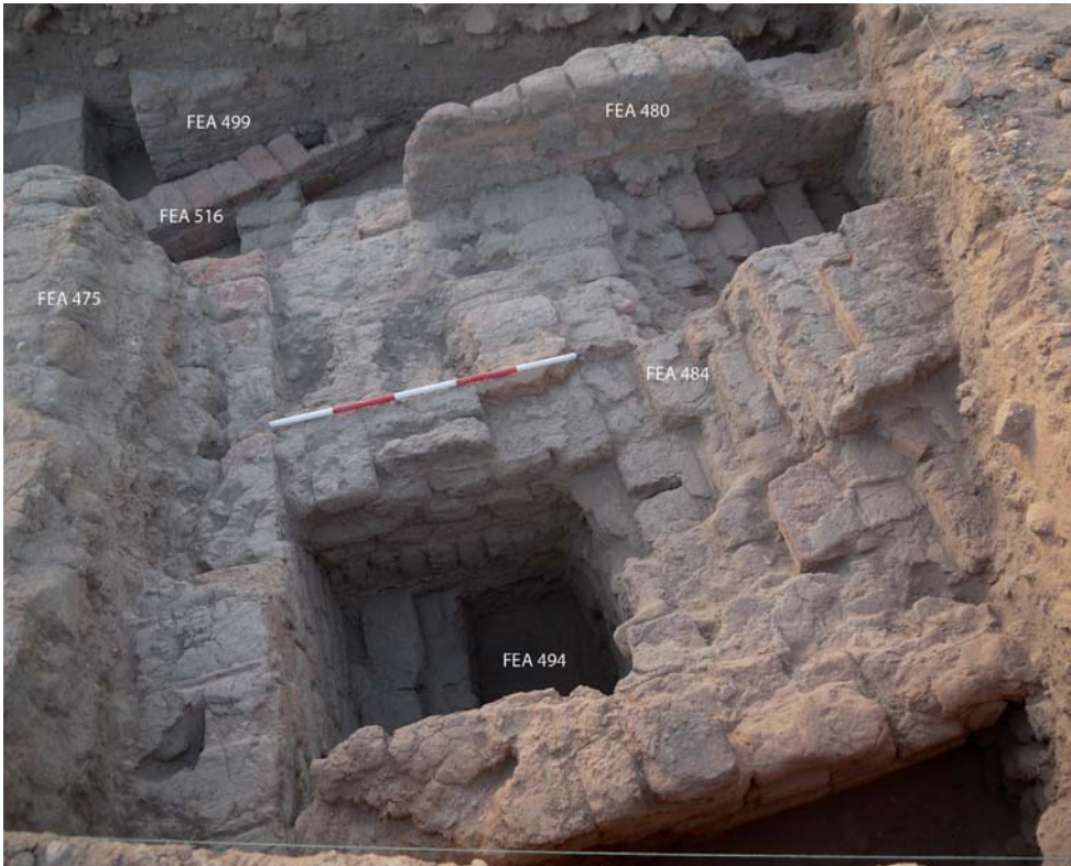
Pl. 1 Section of a staircase between the Typhonium (left) and structure WBN 250 in trench T44; a test pit through the platform can be noted in the centre, a fired brick drainage (FEA 516) can be noted on the top left (Photo: Vlastimil Vrtal).
