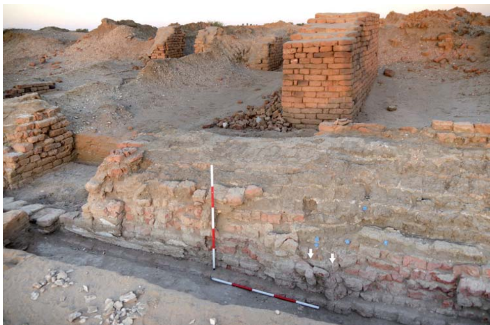
Pl. 2 Section of the exterior wall north of the entrance to WBN 143 (visible on the left); showing position of double torus moulding in situ (marked by arrows). The blue points mark position of special bricks detached from the wall. Protruding foundations can be noted at the foot of the wall (Photo: Vlastimil Vrtal).
