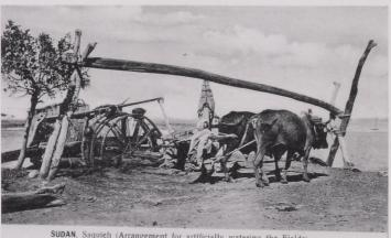
SUDAN. Saquieh (Arrangement for artificially watering the Fields). Saquieh. (Inondation artificielle des champs).
