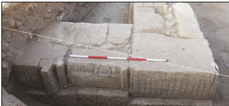
Pl. 12. Reliefs preserved in situ on the southern face of the exterior wall of structure WBN 1100. (Photo: Vlastimil Vrtal).
